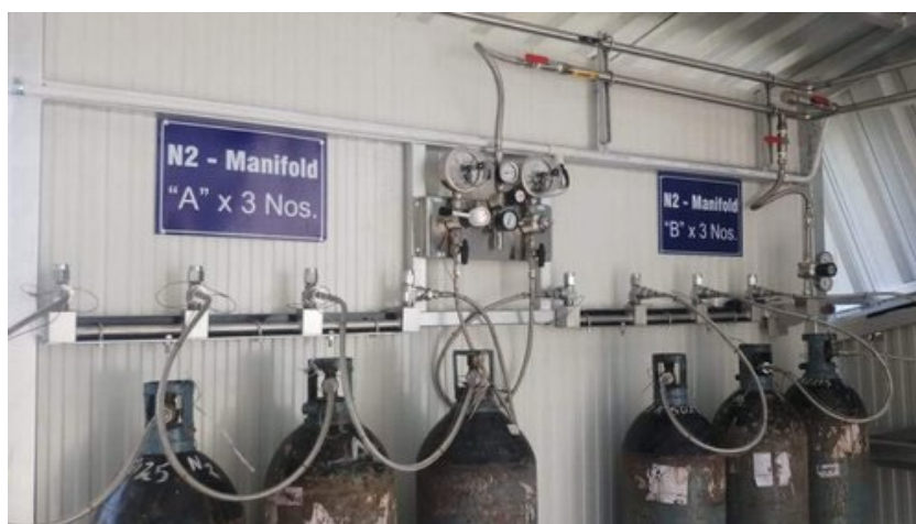
Figure 5. A Manifold Cylinder Bank
